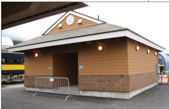
Construction of the new Seward Depot Restroom facility is essentially complete in 2010.
