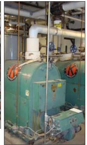
An energy-efficient system (above left) replaces the old boiler system (right).
