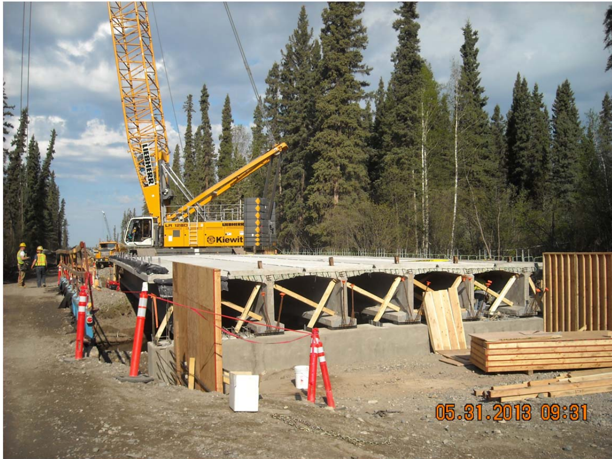
May 31, 2013 – Pile Driver Slough Bridge – All 6 girders set & forming wing walls
