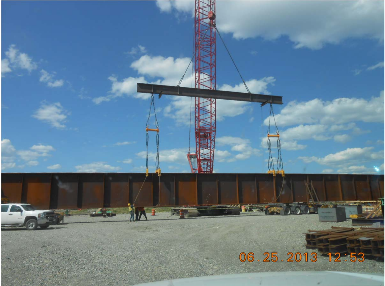
June 25, 2013 – 1 st of the last 24 Girders being Off Loaded on Site
