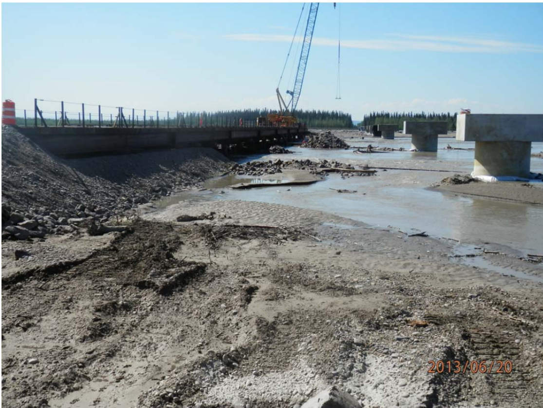
June 20, 2013 – Trestle Bridge and Main Alignment
