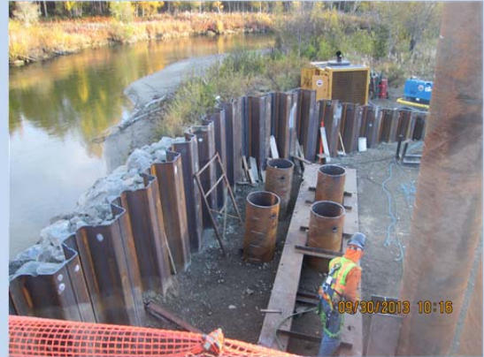
Little Su Bridge South Sheetpile Abutment Work
