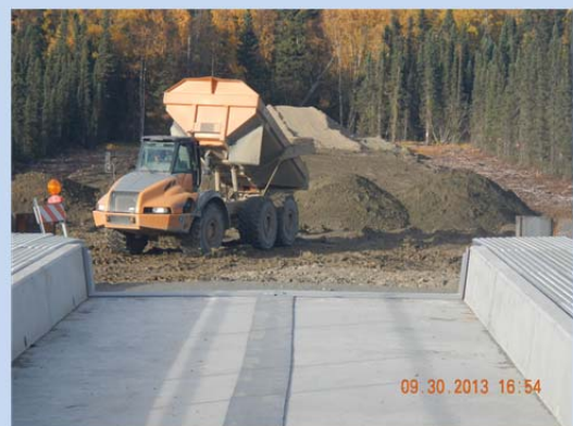
Embankment No. of Completed Baker Farm Bridge
