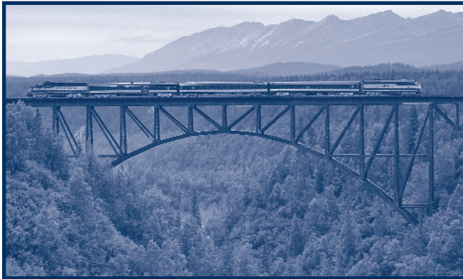
Hurricane Bridge. (Photo by David Blazejewski)
