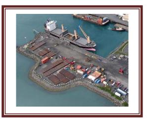
The dock is supported by a sheet pile bulkhead on the west side, a riprap & armor rock fill slope on the east side, and a combination of the two on the south side. It has a series of fenders on the west side where ships dock. A catwalk and mooring dolphin were installed at the end of the dock to aide in berthing of vessels, and the basin adjacent to the new dock was dredged.
