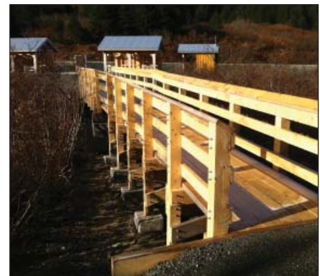
The small bridge over the Placer River.
