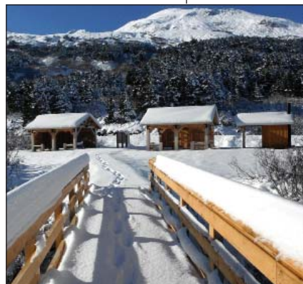
Facility construction complete by winter.
