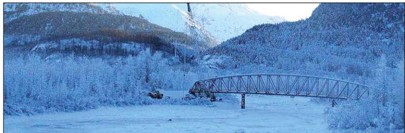
The first of two pedestrian bridges is constructed over Placer River.
