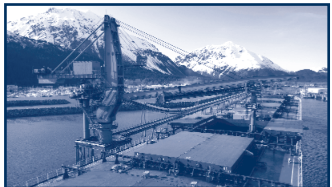
A ship loads at the coal-loading dock, which will be evaluated for use in handling other commodities. (photo by Chris Ahrend)
