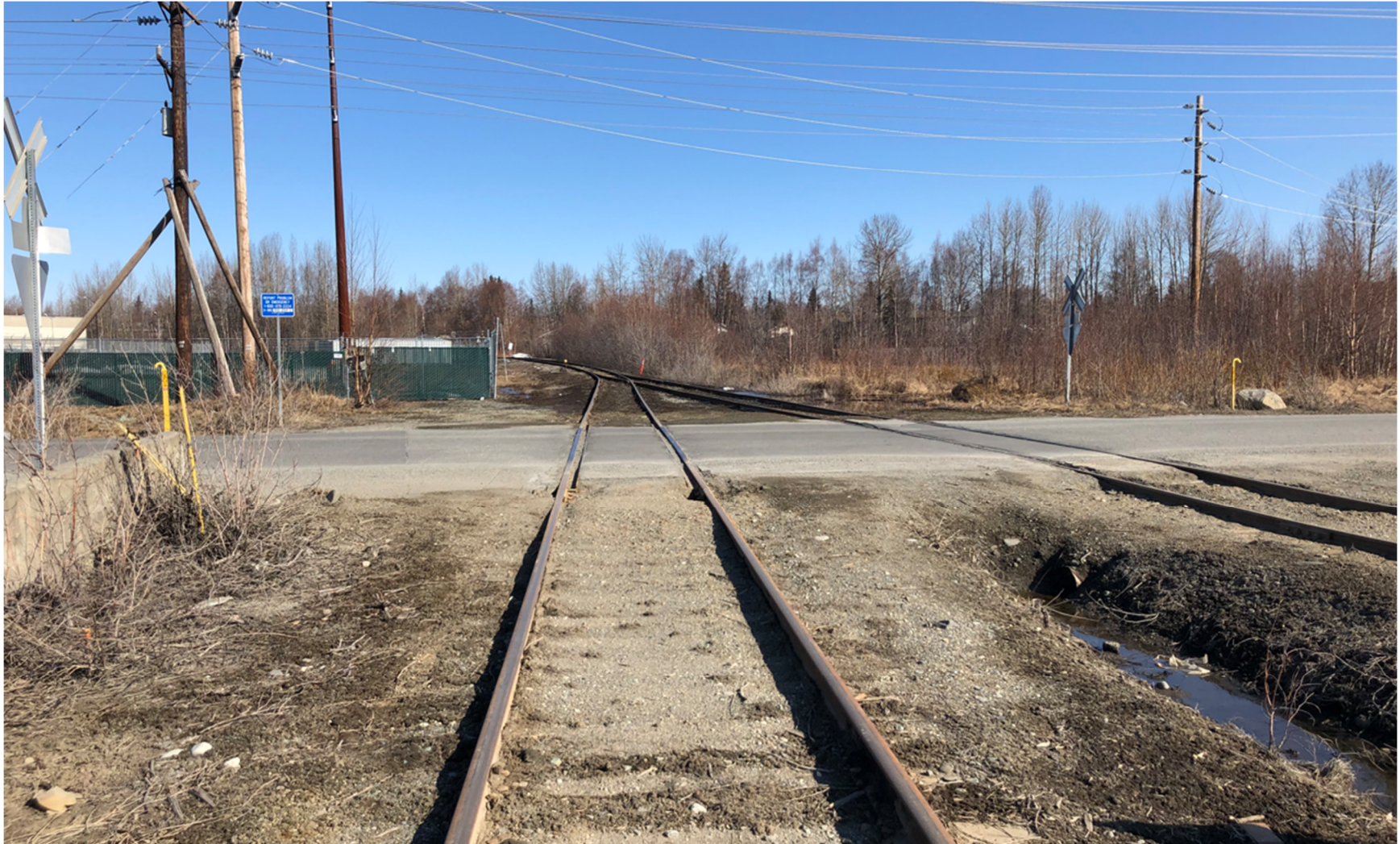
Figure 2 – Electron Drive Crossing Looking North (2022)
