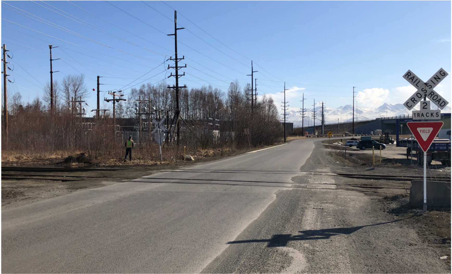
Figure 4 - Electron Drive Crossing Looking East (2022)
