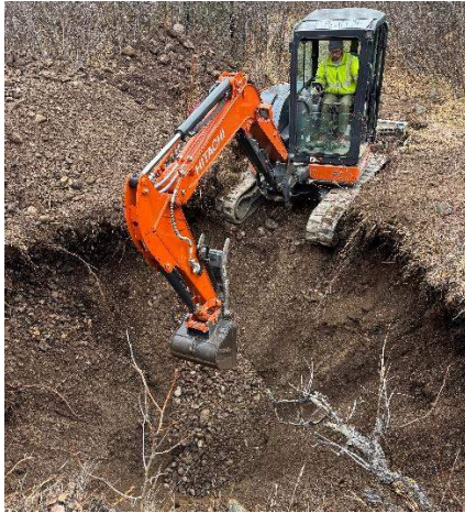
Photo 2.1: Digging TP1, STA 20+00 above CL looking uphill. Bedrock not located in ~15-ft deep pit
