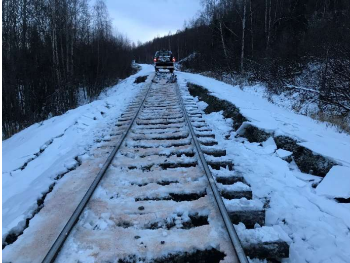
Photo 1: Ice melt placed above the mainline at ≈MP 138.5, looking RR North.
