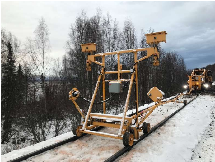
Photo 3: The ET20 realigning and raising the rail at ≈MP138.5, looking RR North-Northwest.
